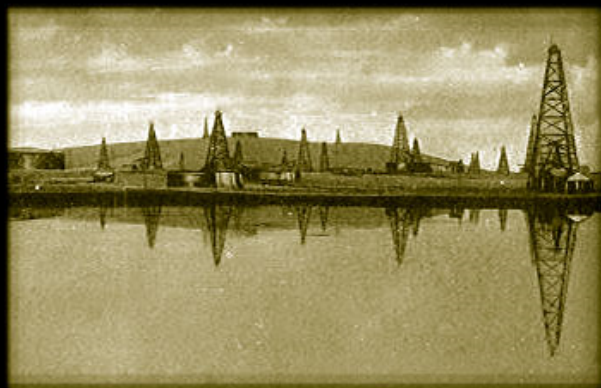
The Lake of Oil - Oil storage before the pipelines were laid was a problem
